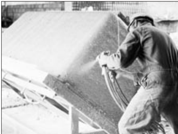
Photograph 5.1 Manual spraying in progress
