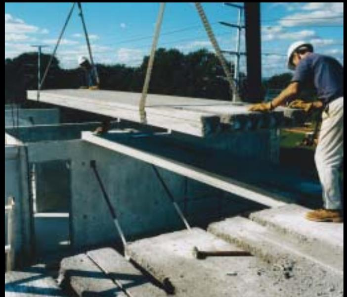
*Hollowcore Floor Planks may be supported on precast walls (above) as detailed in Figure 16 (page 17) or steelwork (below) as detailed in Figure 17 (page 18)*
