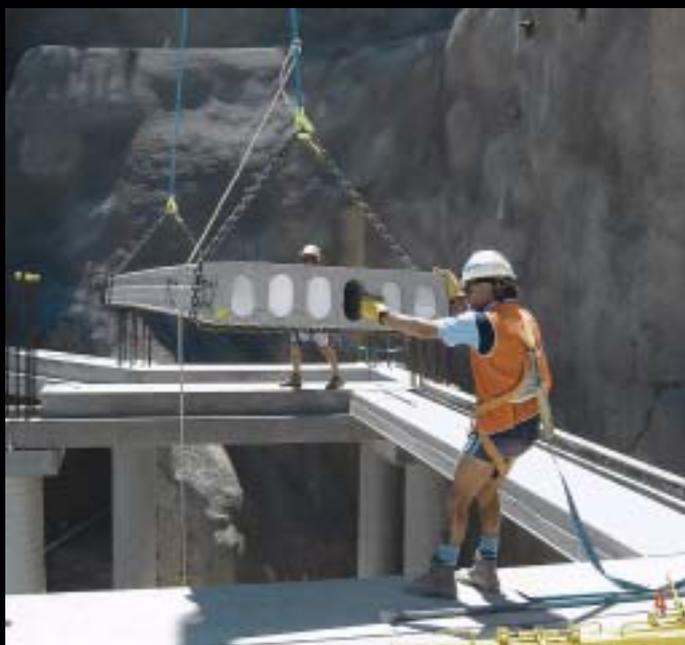
*Hollowcore Floor Planks, as a structural unit:*
