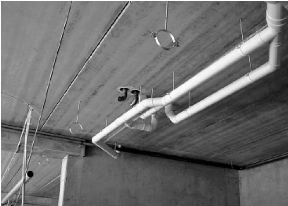
*Penetrations for services and provision for hangers are readily accommodated by hollowcore planks, see Figure 19 (page 20) and Figure 21 (page 21)*
