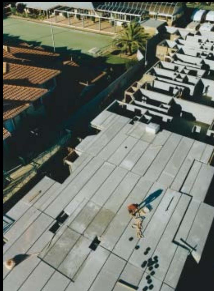
*Hollowcore Floor Planks are ideal for residential construction. They easily accommodate set-downs for wet areas, penetrations for services and step-downs for balconies*
