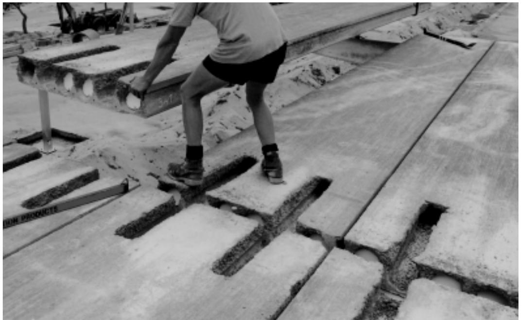
*Core break-outs are used to grout in integrity ties, see Figure 13 (page 13)*
