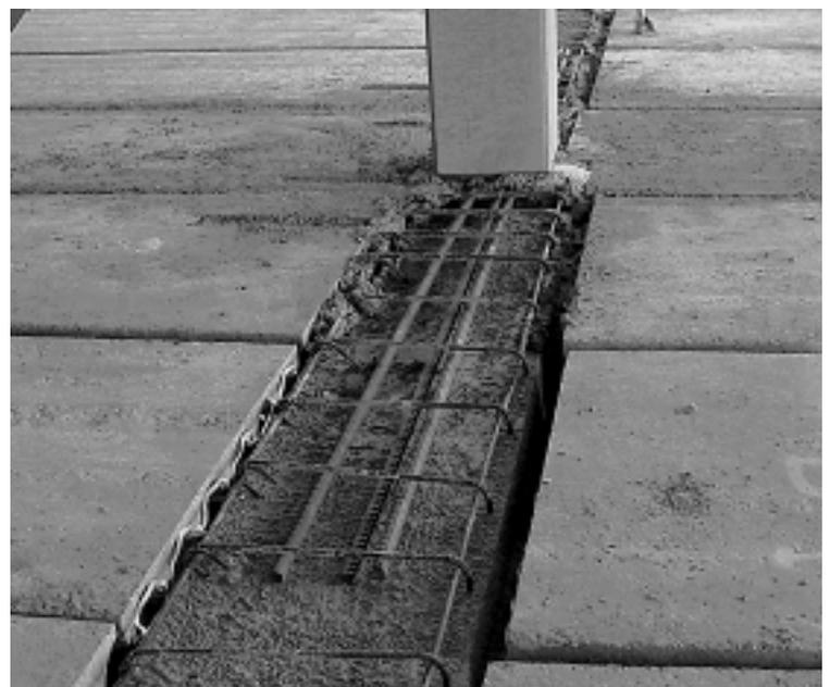
*Typical detail using internal precast support beams and precast columns, see Figure 16 (page 17)*
