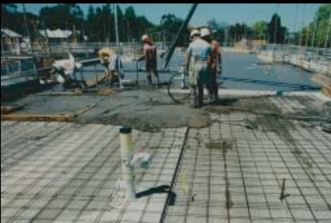
*Topping concrete is often used to produce composite units and a level floor surface, see Figure 1 (page 5)*
