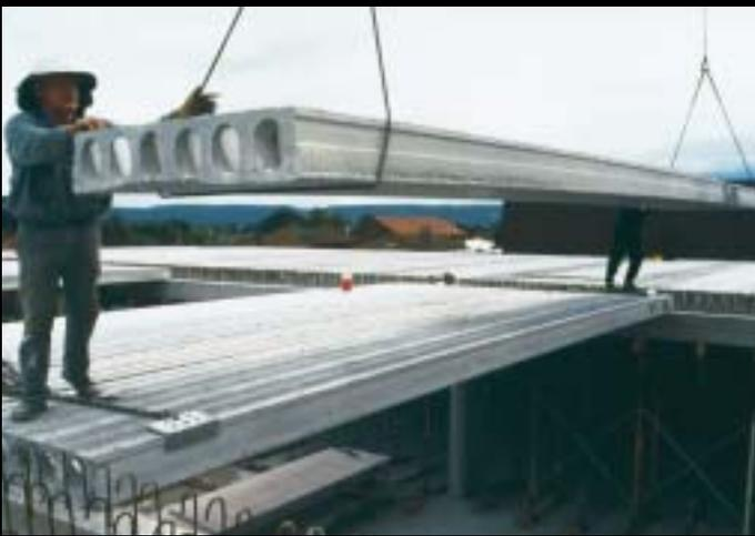
*Hollowcore Floor Planks may be supported on precast beams (above) or masonry walls (below) as detailed in Figure 16 (page 17)*
