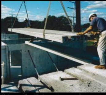
Hollowcore Floor Planks may be supported on precast walls (above) as detailed in Figure 16 (page 17) or steelwork (below) as detailed in Figure 17 (page 18)
