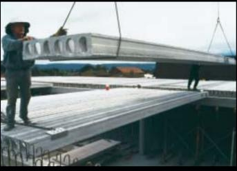
Hollowcore Floor Planks may be supported on precast beams (above) or masonry walls (below) as detailed in Figure 16 (page 17)
