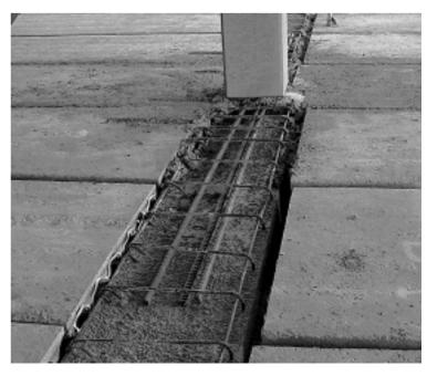
Typical detail using internal precast support beams and precast columns, see Figure 16 (page 17)
