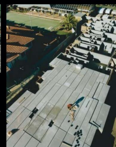
Hollowcore Floor Planks are ideal for residential construction. They easily accommodate set-downs for wet areas, penetrations for services and step-downs for balconies
