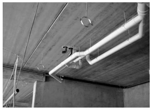
Penetrations for services and provision for hangers are readily accommodated by hollowcore planks, see Figure 19 (page 20) and Figure 21 (page 21)
