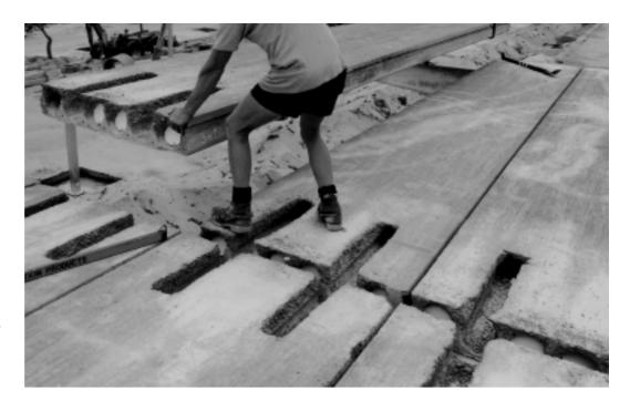
Core break-outs are used to grout in integrity ties, see Figure 13 (page 13)
