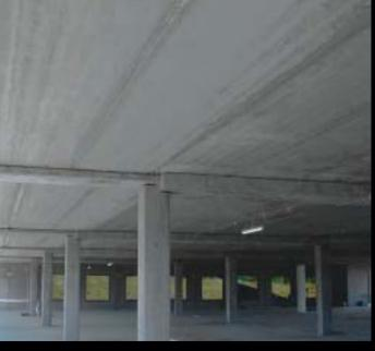
Hollowcore Floor Planks, as a floor system, provide:
