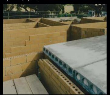
Topping concrete is often used to produce composite units and a level floor surface, see Figure 1 (page 5)
